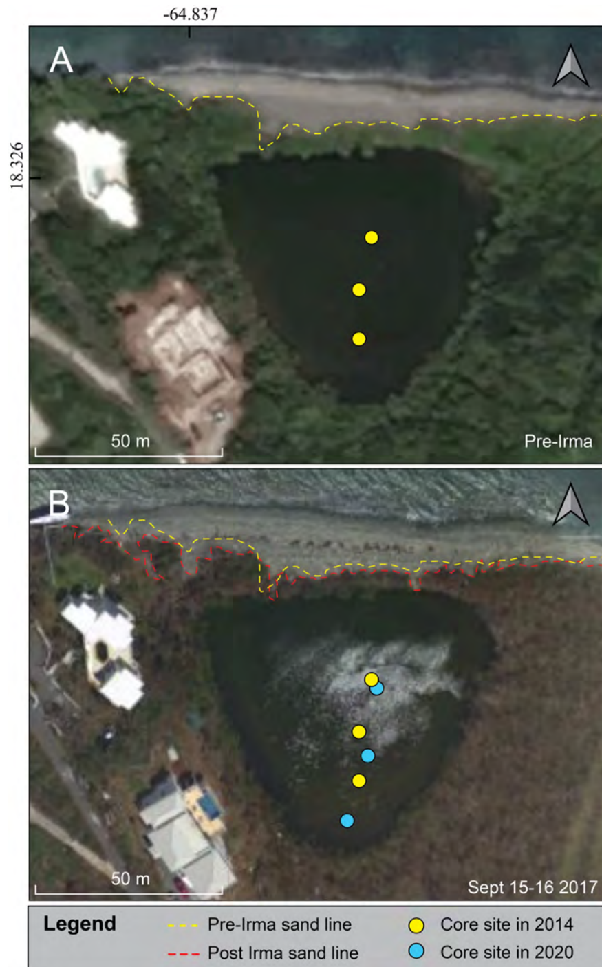
Figure 8. Before (A) and after (B) Hurricane Irma imagery of Cabrita Pond on St. Thomas (from National Geodetic Survey, 2021). On B, note several small overwash fans formed in areas of previous fans and may have reached the edge of the pond but otherwise there appeared to be little effect on the pond.
